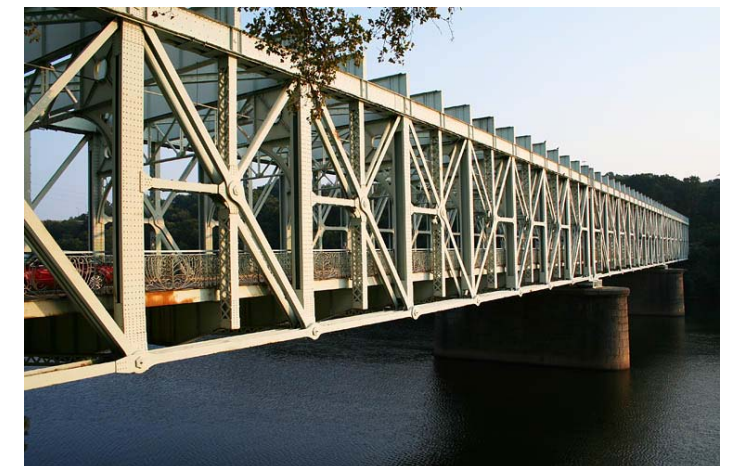
The Falls Bridge
